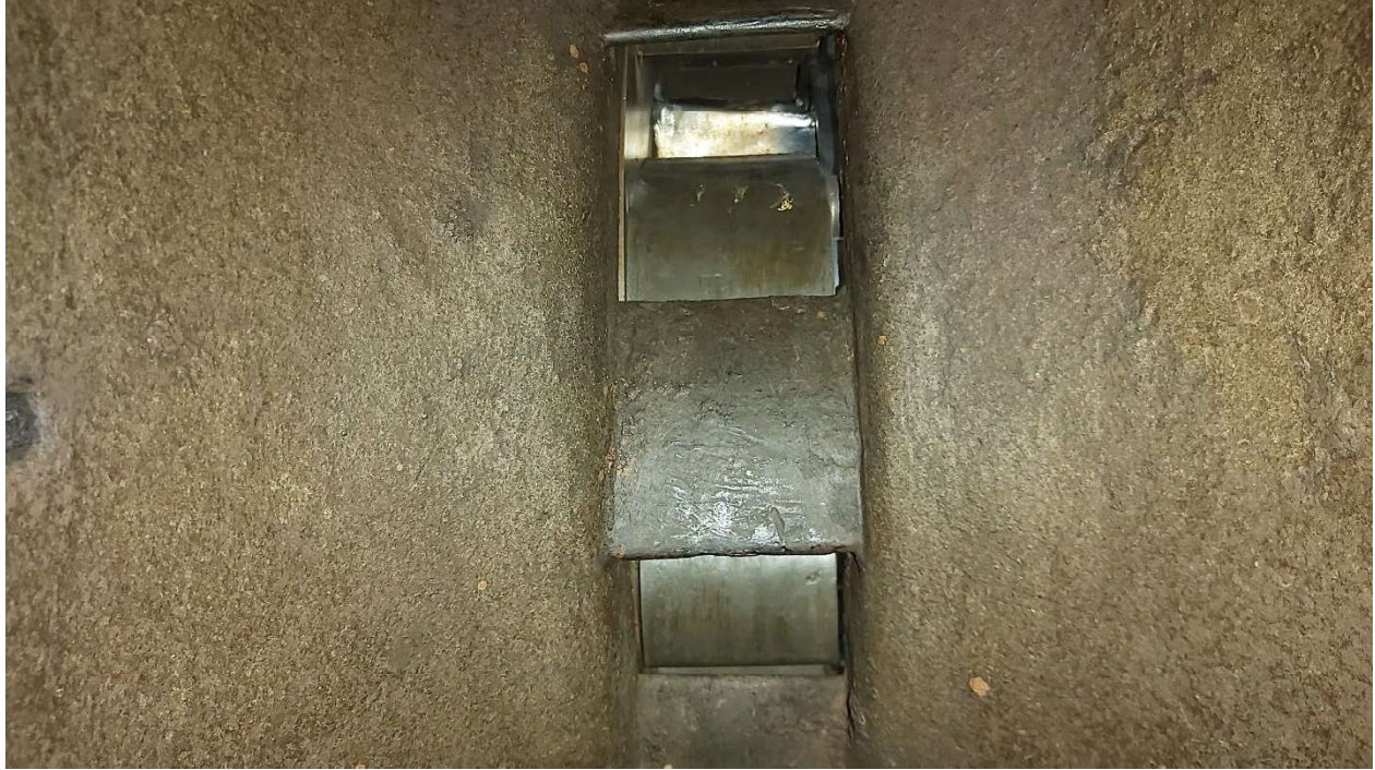
Figure 9: Scroll Case and Stay Vane High Friction Condition
